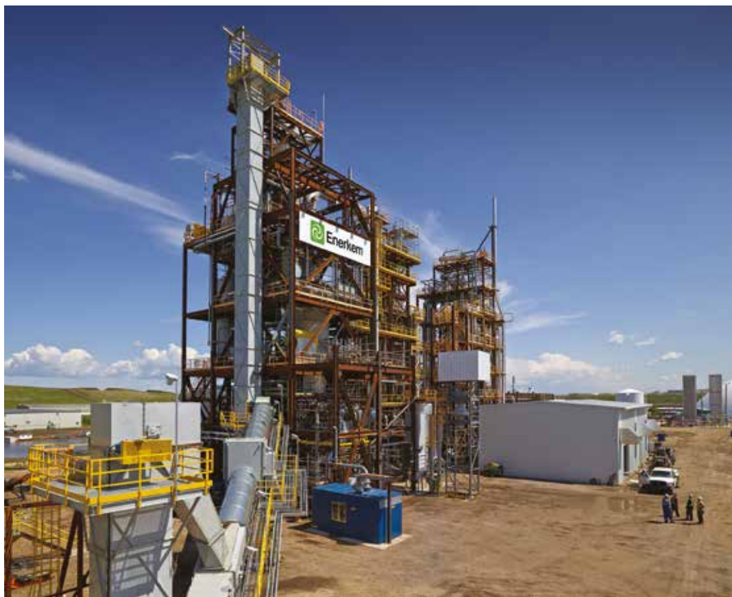
Enerkem's biofuels facility in Alberta, Canada
